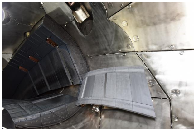
Fig. 7: Final assembled scraper element, piggyback mounted on wall shield elements. In the background: the graphite target elements of the horizontal and vertical divertor and some adjacent baffle modules.
