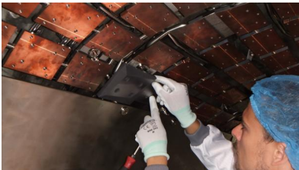
Fig. 8: Assembly of the first out of 8000 graphite tiles at W7-X
