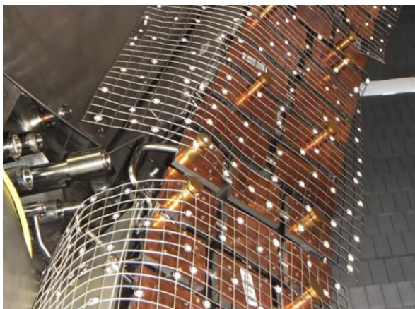
Fig. 4: Reference point system installed on cooling structures. The reference points (white points) are fixed in arbitrary distances at a stainless steel wire grid
