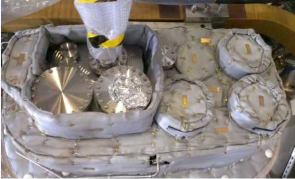
Fig. 5 Typical insulation and baking mats at port flanges
