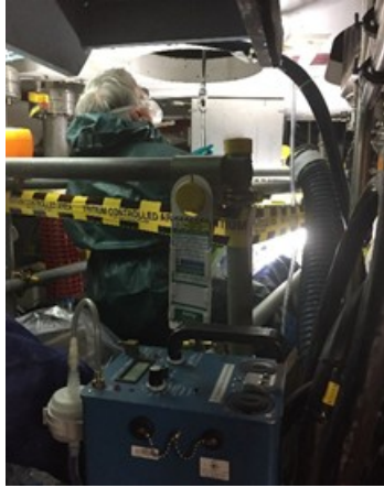
Figure 2 - Person #1 removing Drain flange bolts.
