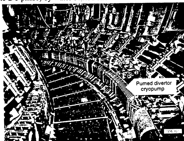
Fig. 1 The in-vessel cryopump for the JET pumped divertor as installed at the bottom of the torus before the installation of the high heat flux elements
