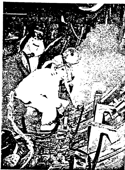
Fig.5: An in-vessel operator wearing a full pressurised suit and using the 100 bar boron carbide grit water gun to clean the JET vessel
