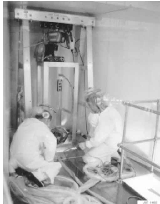
Fig 1 Suited personnel preparing the hoist in the NIB access cabin
