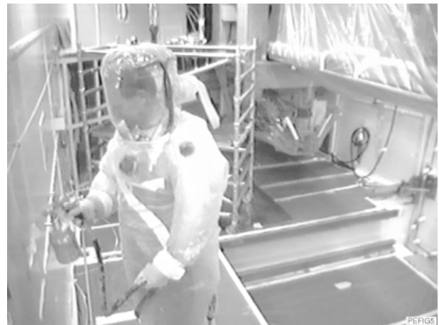
Figure 5. Application of the sacrificial strippable coating by spray gun.
