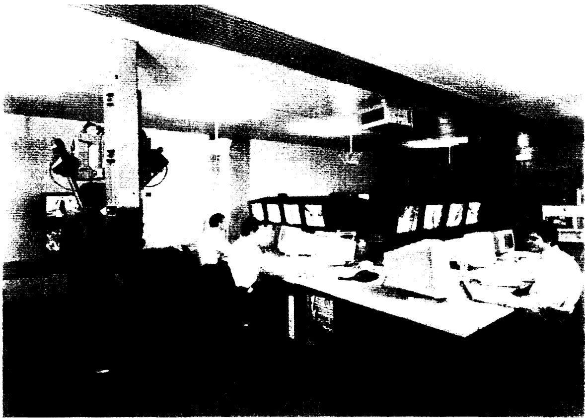
Figure 1 Remote Handling Control Room
