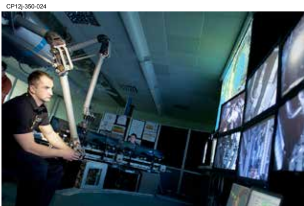
Figure 1: JET Remote Handling Control Room.
