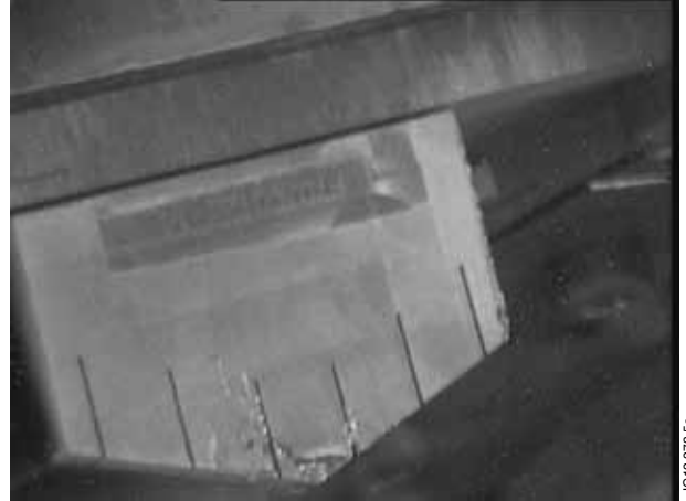
Figure 5: Disruption damage to the upper dump plate tiles.
