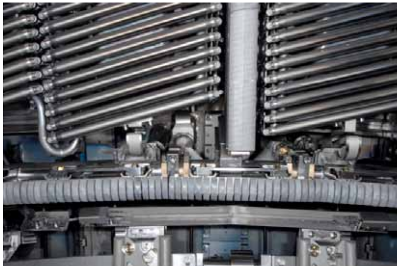
Figure 2: Close view of an A2 antenna's lower part showing Be-screen bars, part of the new Be septa and horizontal bars.
