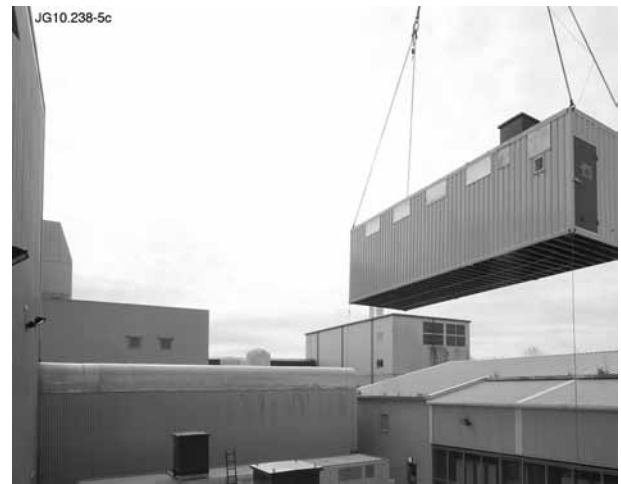
Figure 2: Installation of the last power Unit of ERFA.
