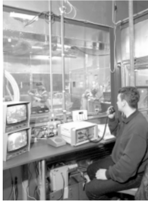
Fig.3: Beryllium handling facilities control station.
